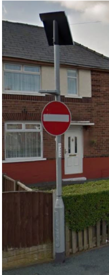
Solar powered sign
